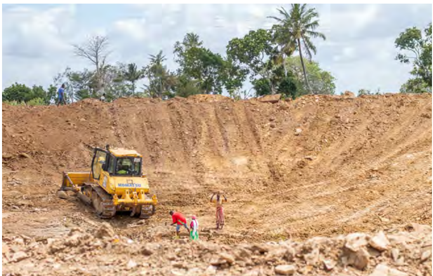
Miyani dam inprogress
